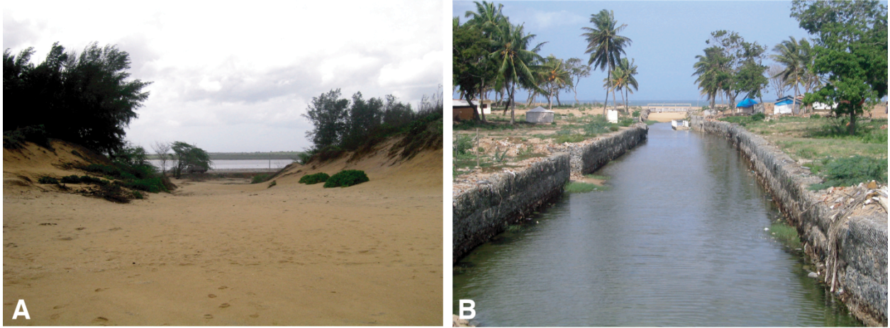
Figure DR6. A: Artificial cut created in 1998 to divert flooding on the southern coast of Karagan Lagoon (Stanzel et al., 2002). Photo is from the southern beach looking north with Karagan Lagoon in the background. B: The natural mouth of the lagoon runs through the town of Hambantota and was reinforced in 1998 with concrete walls to control the flow of water and prevent the town from flooding. Photos taken in August 2005.
